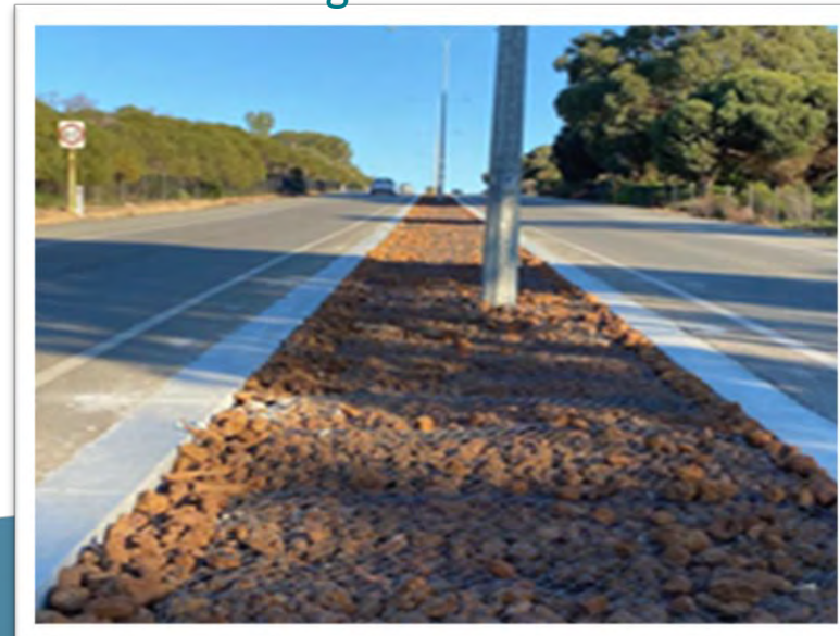
Road Drainage Upgrade - Gabion cages max infiltration
