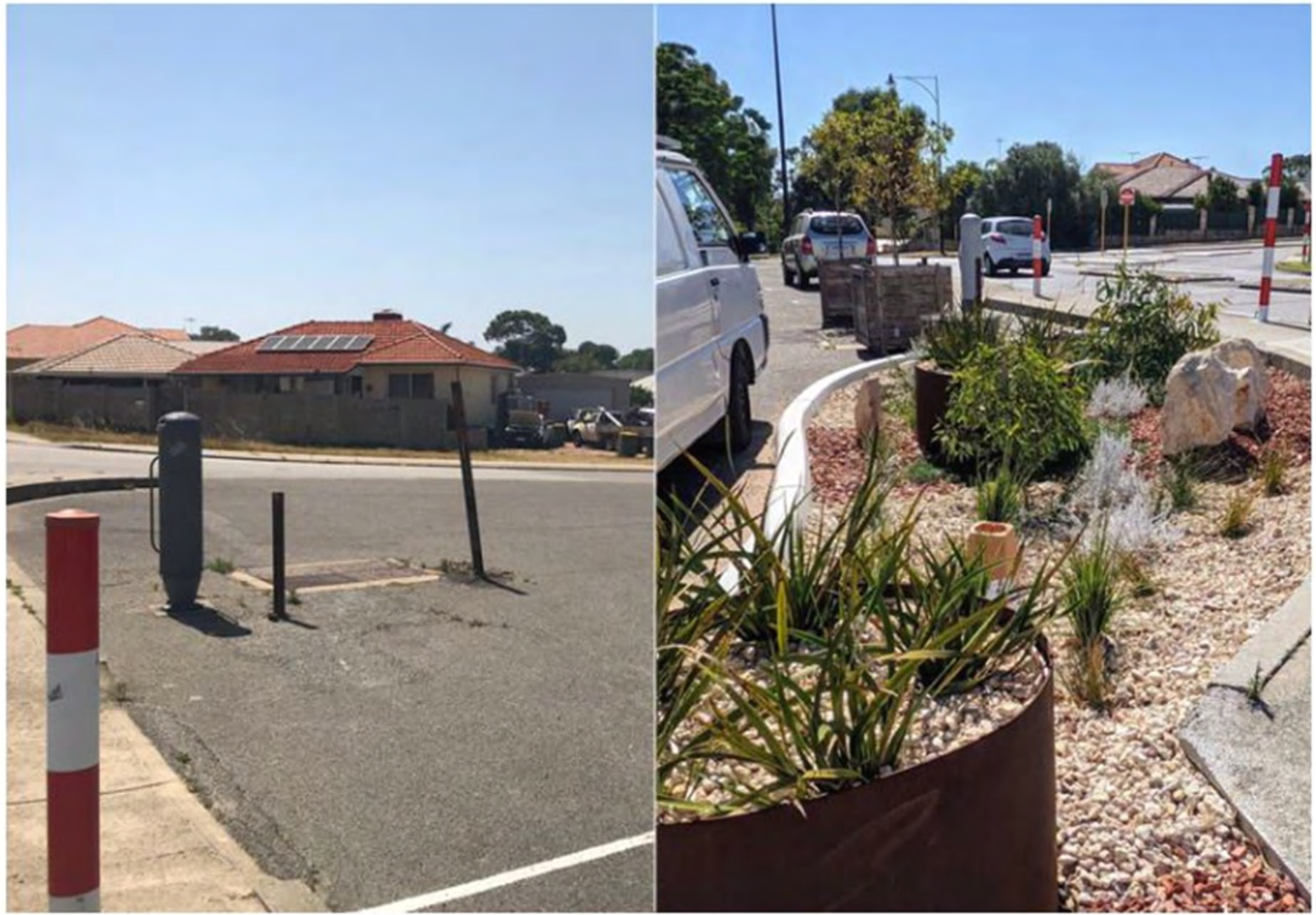
Before and after: The car park has been converted to include a water sensitive urban designed garden and mixed use space.
