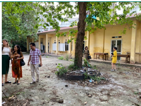
HUCE C4 disused buildings to be refurbished incorporating NBS
